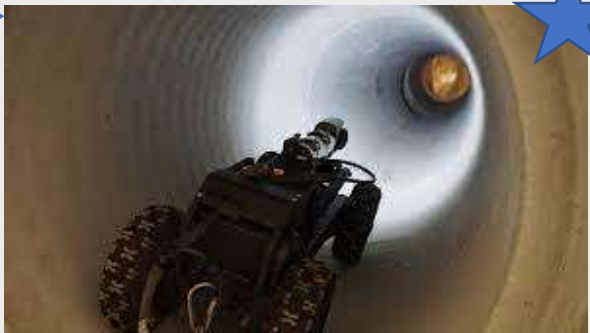
Inspections - Storm and wastewater pipelines
