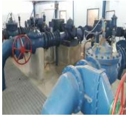
Water Loss Control Program 10% Non-revenue water loss (<15%)
