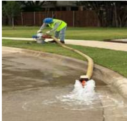
Flushed dead end lines 475 times (4.8 MG)
