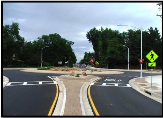
Example of a modern roundabout approach
