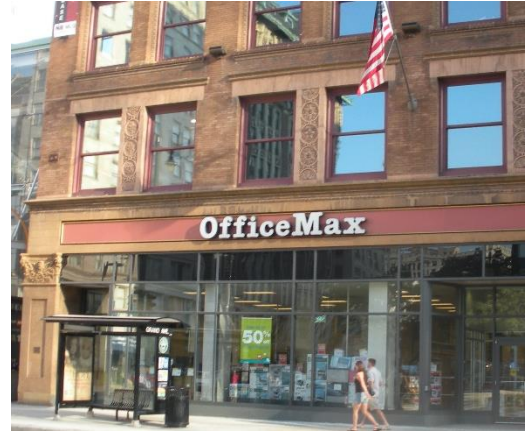
Example of a Wall Sign
