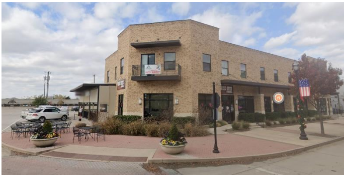
Corner buildings provide a setback with a corner entrance
