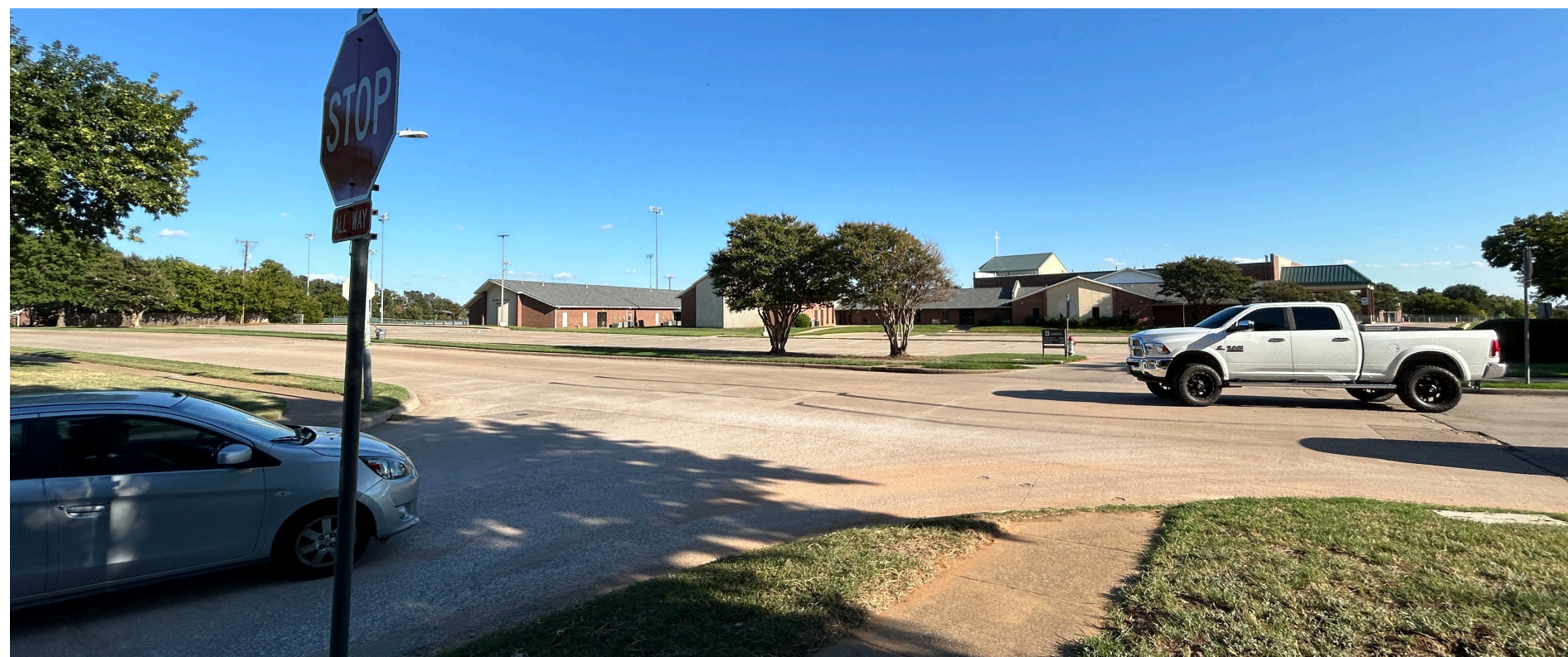
Inadequate crossing and sidewalk connection at the intersection of Meadowview Drive and Vistaview Drive.
