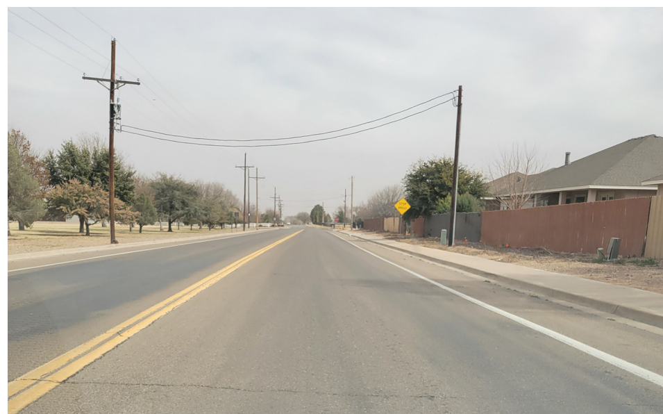
Shared bike lane and parking lane on Mescalero Road in Roswell, New Mexico
