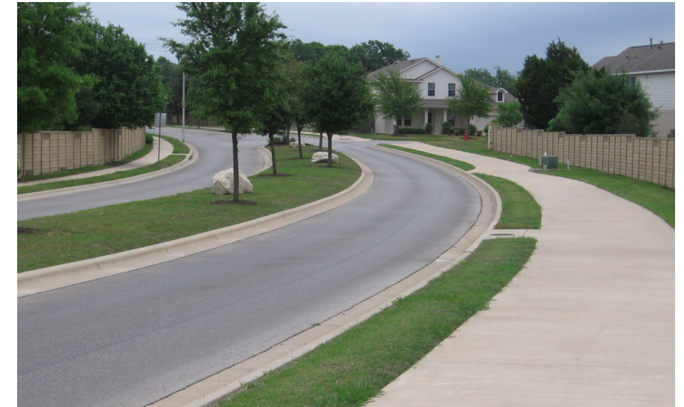
Shared-use path on one side of E. Park Street in Cedar Park, Texas
