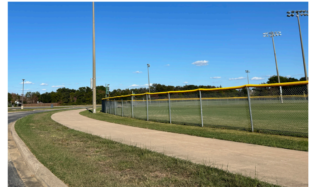
Exhibit 27. Shared-use path in the Corinth Community Park
