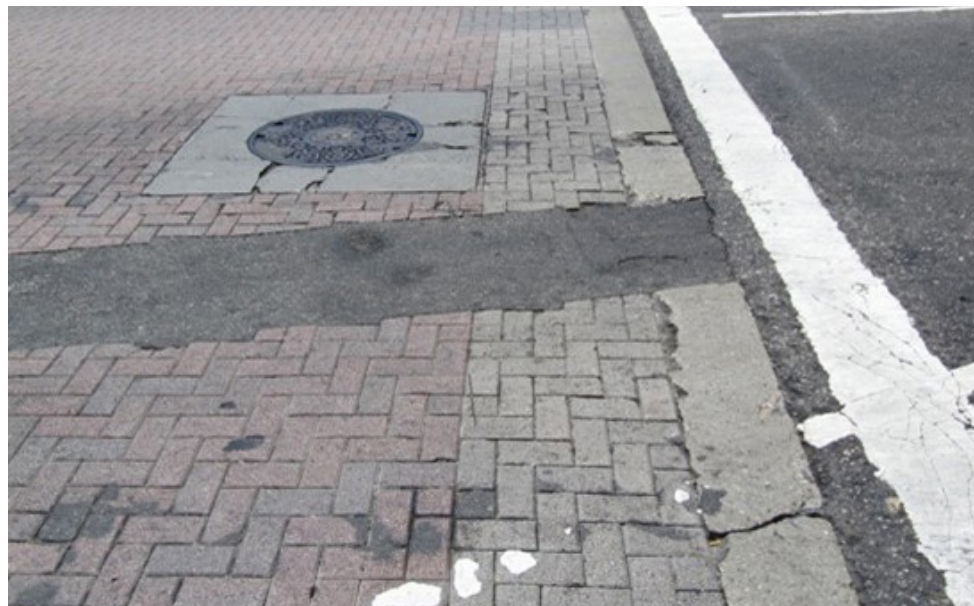
Decorative crosswalk treatments made of distinctive materials can become uneven over time. (Credit: Ryan Snyder)
