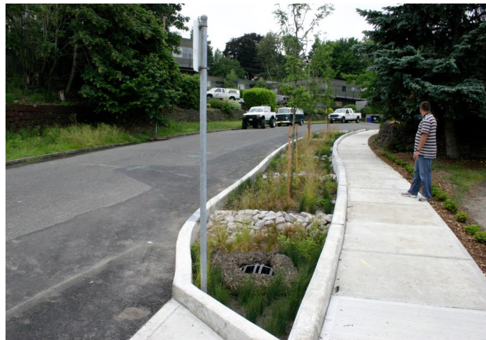
Mid-block curb extension with bioswale. (Credit: Brad Lancaster)
