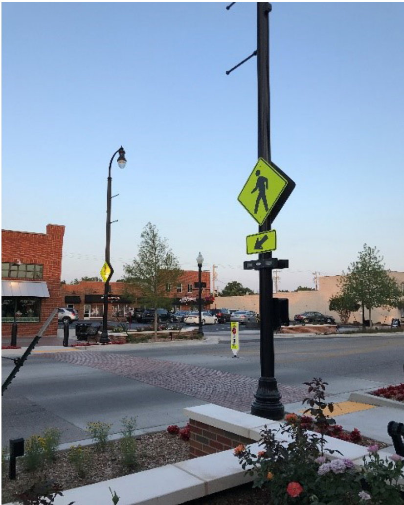
Rectangular rapid-flash beacon in Broken Arrow, Oklahoma.
