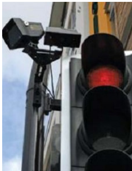
Automated pedestrian sensor used for a PUFFIN signal. (Source: FHWA)
