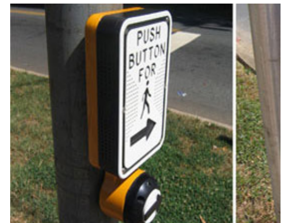
Accessible pedestrian signal. (Credit: Guidelines for Accessible Pedestrian Signals)
