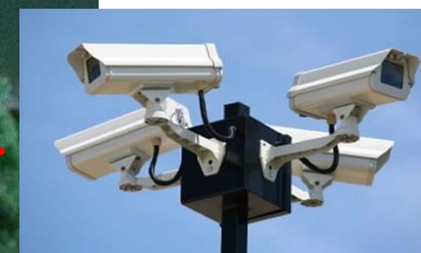
Typical Camera on on Light Posts
