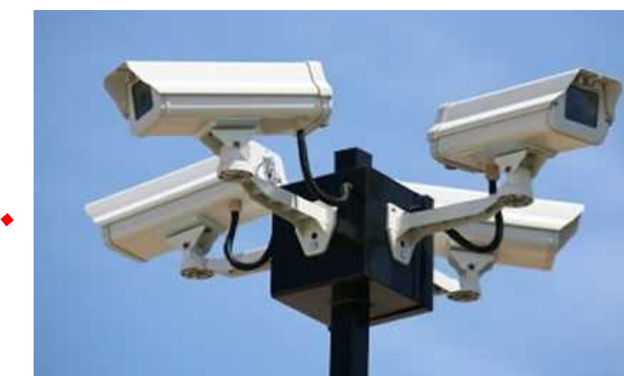
Typical Camera on on Light Posts
