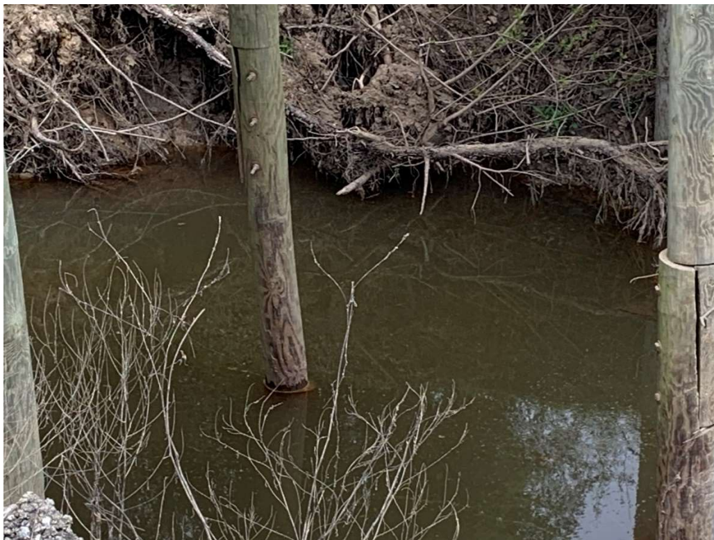
Oxbow bridge support separation
