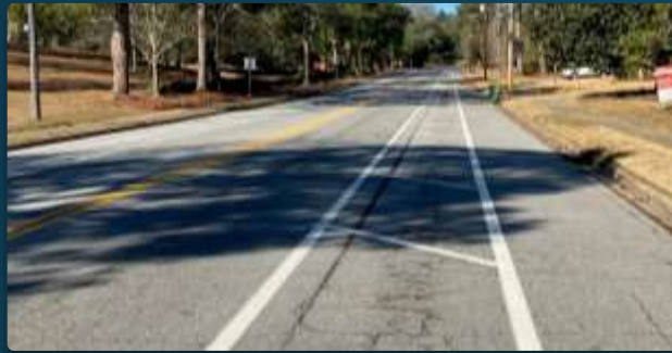
Edgewood Road Striping
