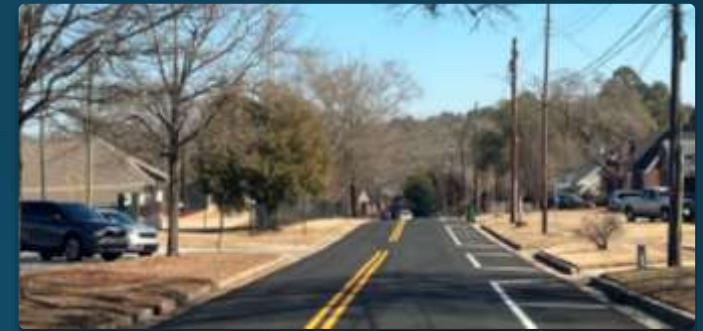
32 nd Street Resurfacing/Striping
