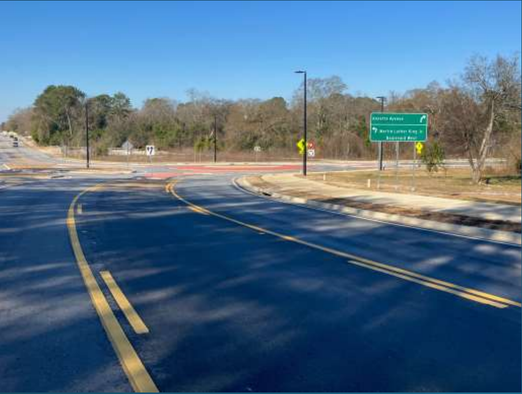
Phase I Roundabout
