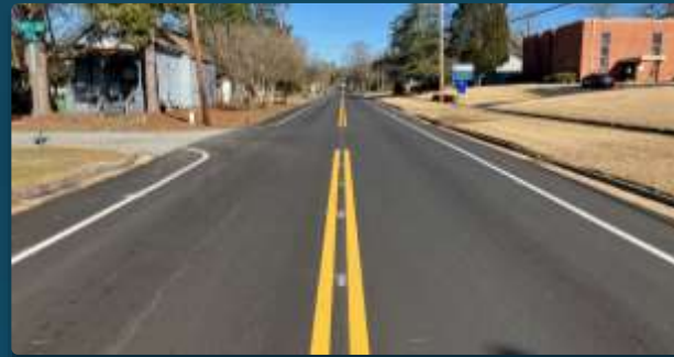
12 th Avenue Resurfacing/Striping
