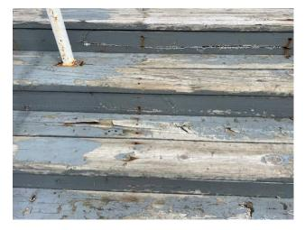
Wood treads contain exposed nails and splintered
