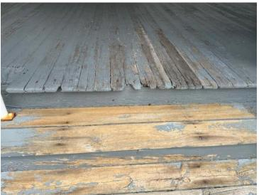
Tread wear observed near the top of both staircases
