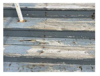
Wood treads contain exposed nails and splintered
