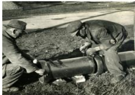
SETTING A NEW LATERAL.—1950's.
