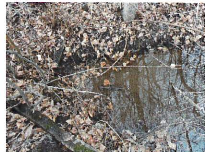
North end of pipe into Wetland #3
