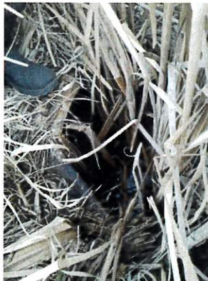
Closeup of inflow of culvert on south side of Highway 2.
