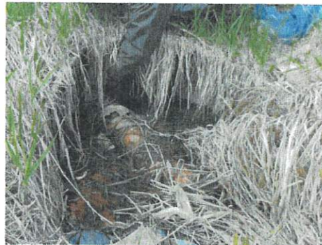
North side of culvert which passes under Hwy 2
