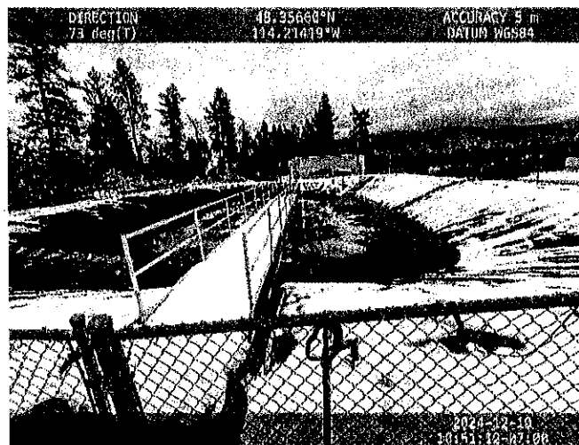
Emergency storage pond.
