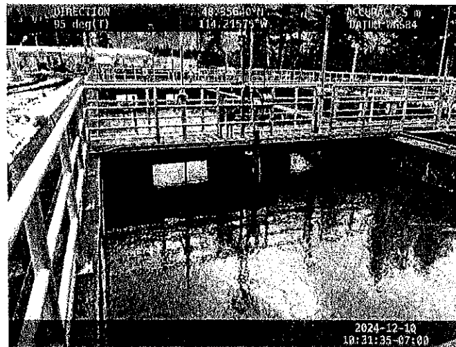
Overlooking the bioreactor (anaerobic zone).
