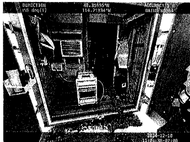
Camera trailer used for maintenance of the SSCS.
