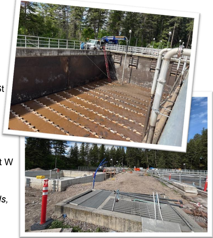
Wastewater Treatment Plant Expansion and Modernization Project
