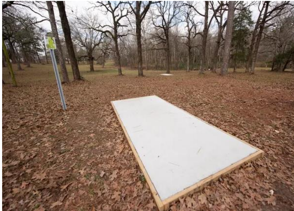
Concrete tee pad
