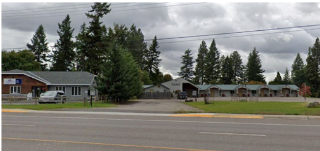
PROJECT SITE ACCESS VIA HIGHWAY 2
