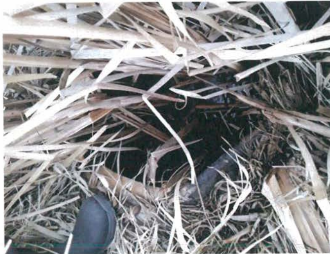
South side of culvert which passes under Hwy 2
