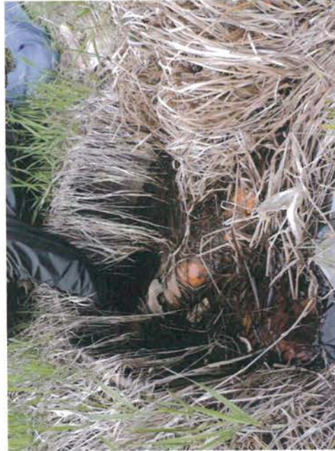
North side of culvert which passes under Hwy 2
