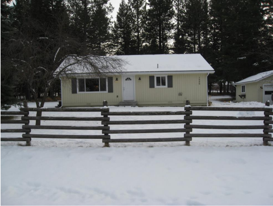
View of Existing home located at 1550 14 th Street EN.
