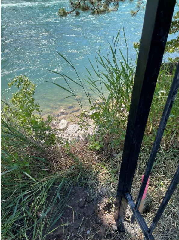
Installed on top of bluff as structurally feasible
