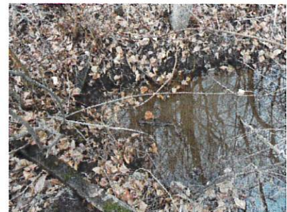
North end of pipe into Wetland #3
