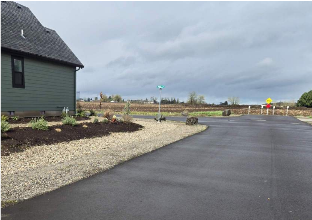
Figure 57: Coburg Creek roadside stormwater facilities on N. Coleman St. in 2024.
