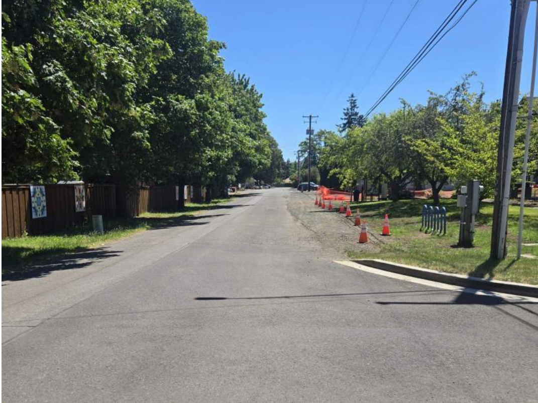
Figure 24: Construction of Pavilion Park improvements including an infiltration trench began in spring of 2024 and completed in mid-2025.
