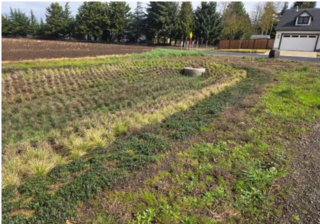
Figure 20: Downstream end of city-owned swale located north of Coburg Creek subdivision, showing overflow to Muddy Creek tributary in 2024.
