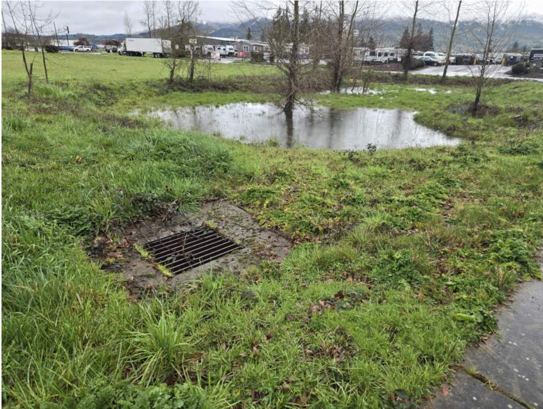
Figure 22: Stormwater pond at south end of Coburg Industrial Way.
