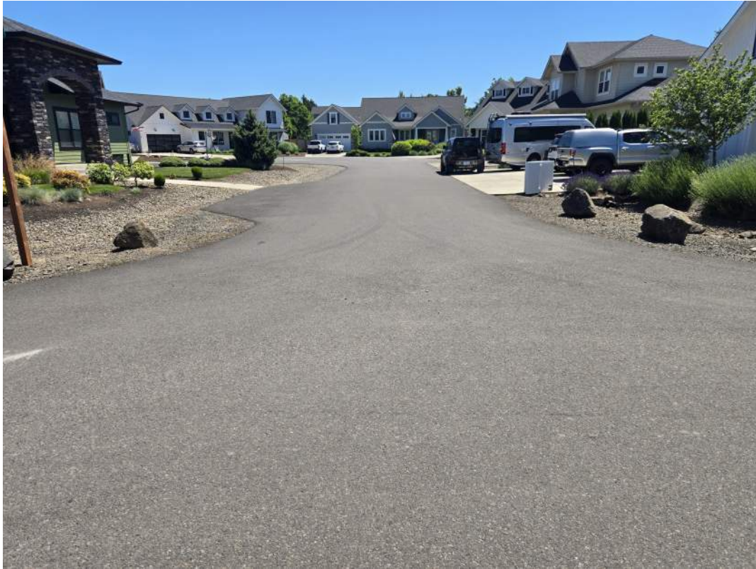
Figure 49: Hatfield Estates roadside stormwater facilities in 2024.
