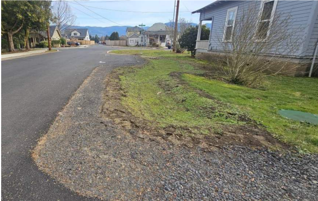
Figure 29: E. Macy St. completed storm facility at construction completion in 2024.
