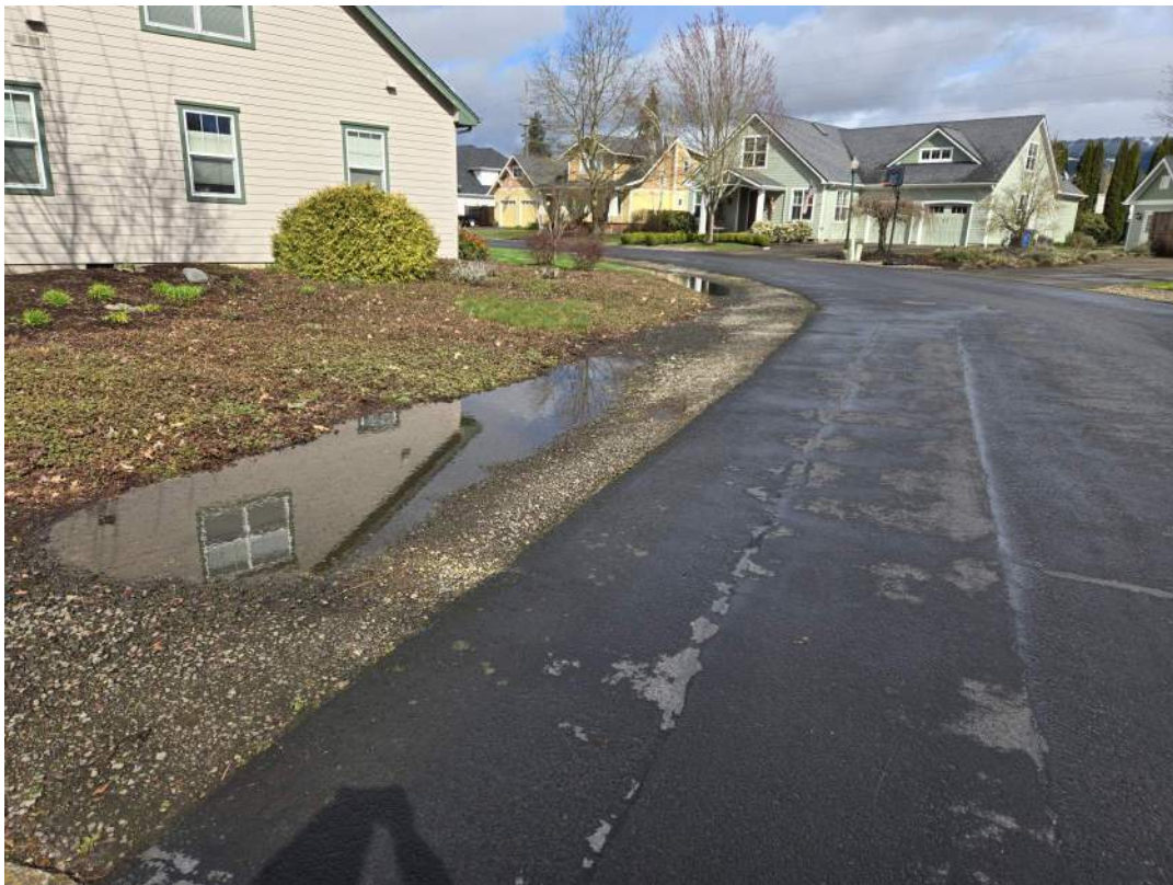
Figure 87: Austin St. infiltration deficiency in 2024.
