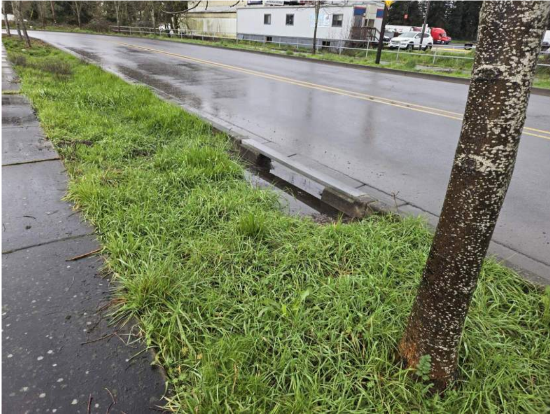
Figure 90: Coburg Industrial Way curb inlet in 2024.
