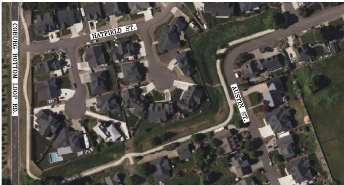
Figure 1: Detention swales in NW of Coburg, with overflow draining into tributary to Muddy Creek.
