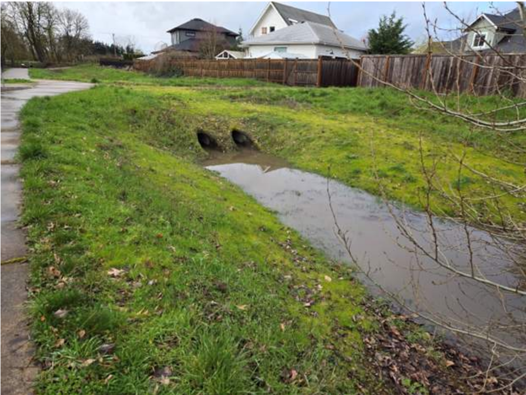
Figure 17: Downstream end of city-owned swale adjacent to Hatfield Estates in 2024.
