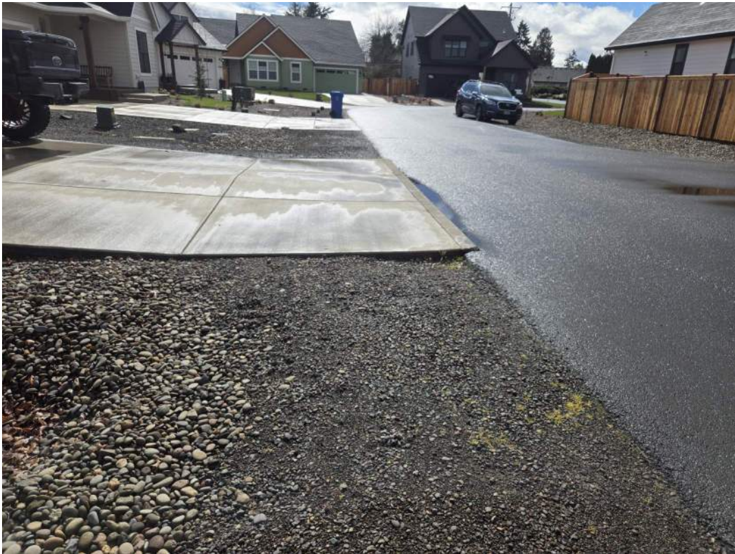
Figure 56: Coburg Creek roadside stormwater facilities along Coburg Creek Rd. in 2024.
