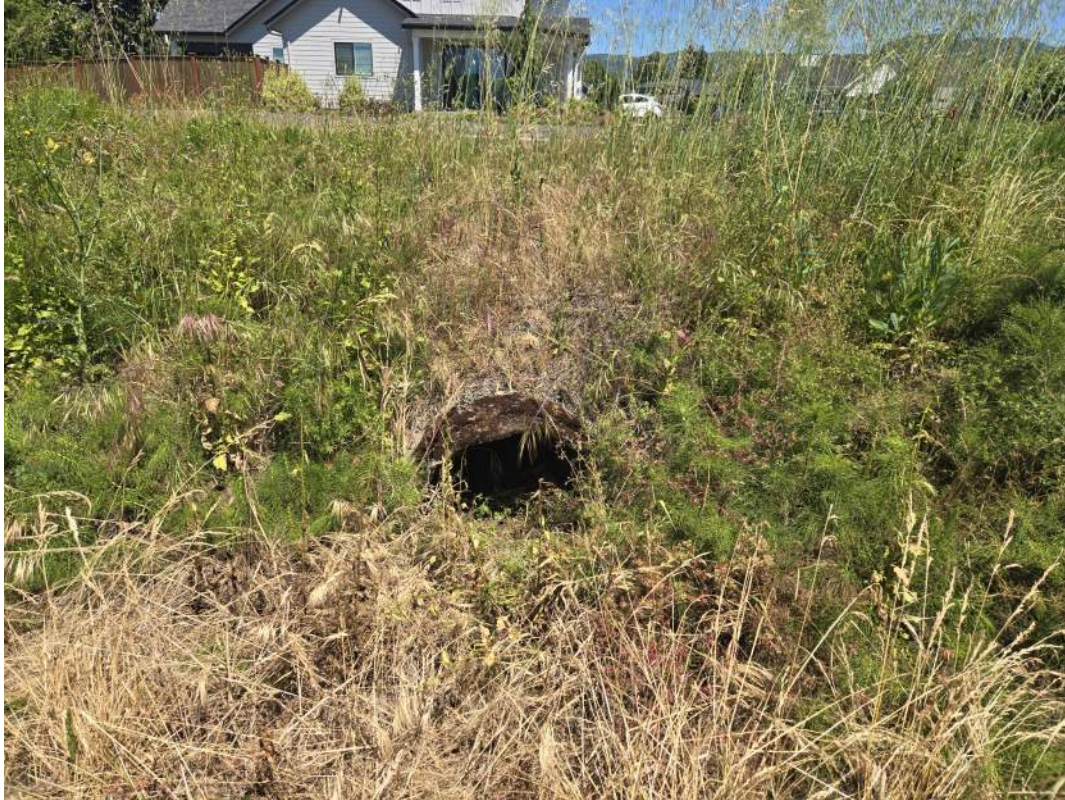
Figure 51: Outlet from the Hatfield Estates stormwater system in 2024, draining to the Mill Slough.
