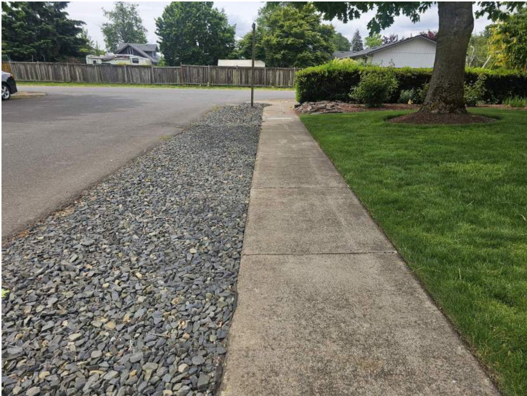
Figure 47: Reconstructed infiltration trench in 2024 on Rustic Ct.
