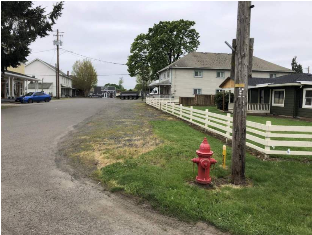
Figure 42: North side of Mill Street in 2018 prior to 2018 reconstruction project.
