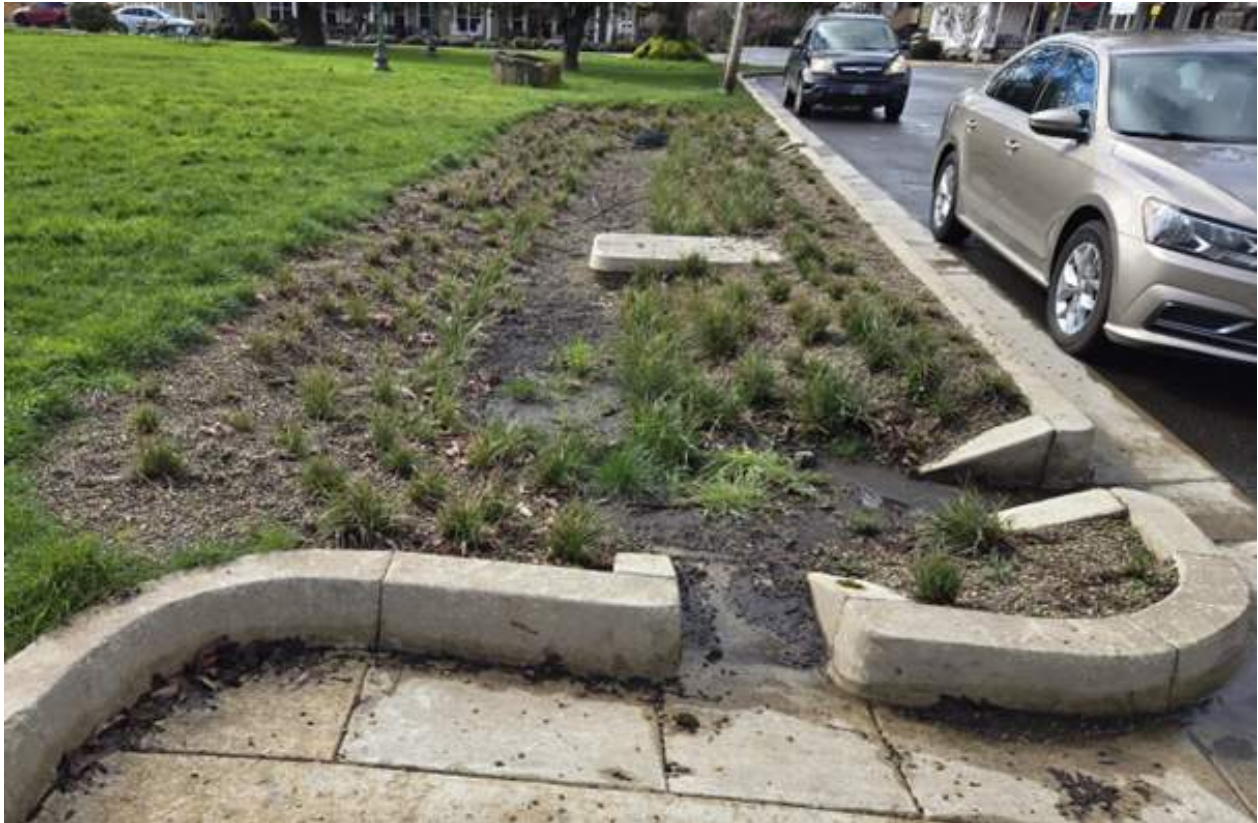
Figure 39: McKenzie St. rain garden in 2024, included in the 2022 reconstruction project.
