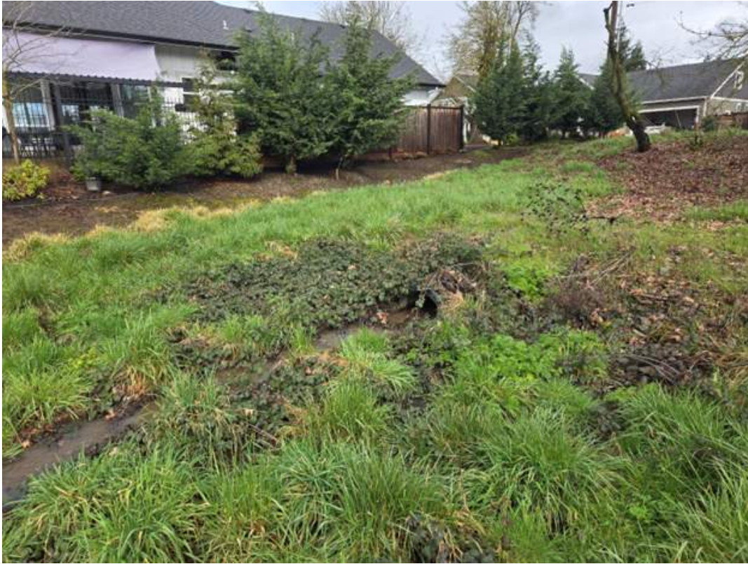
Figure 16: Upstream end of city-owned swale adjacent to Hatfield Estates in 2024.
