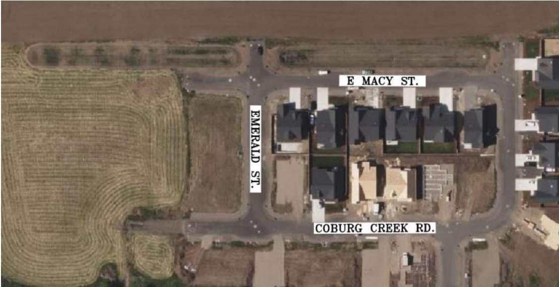
Figure 2: Detention swales in NW Coburg, with overflow to Mill Slough.
