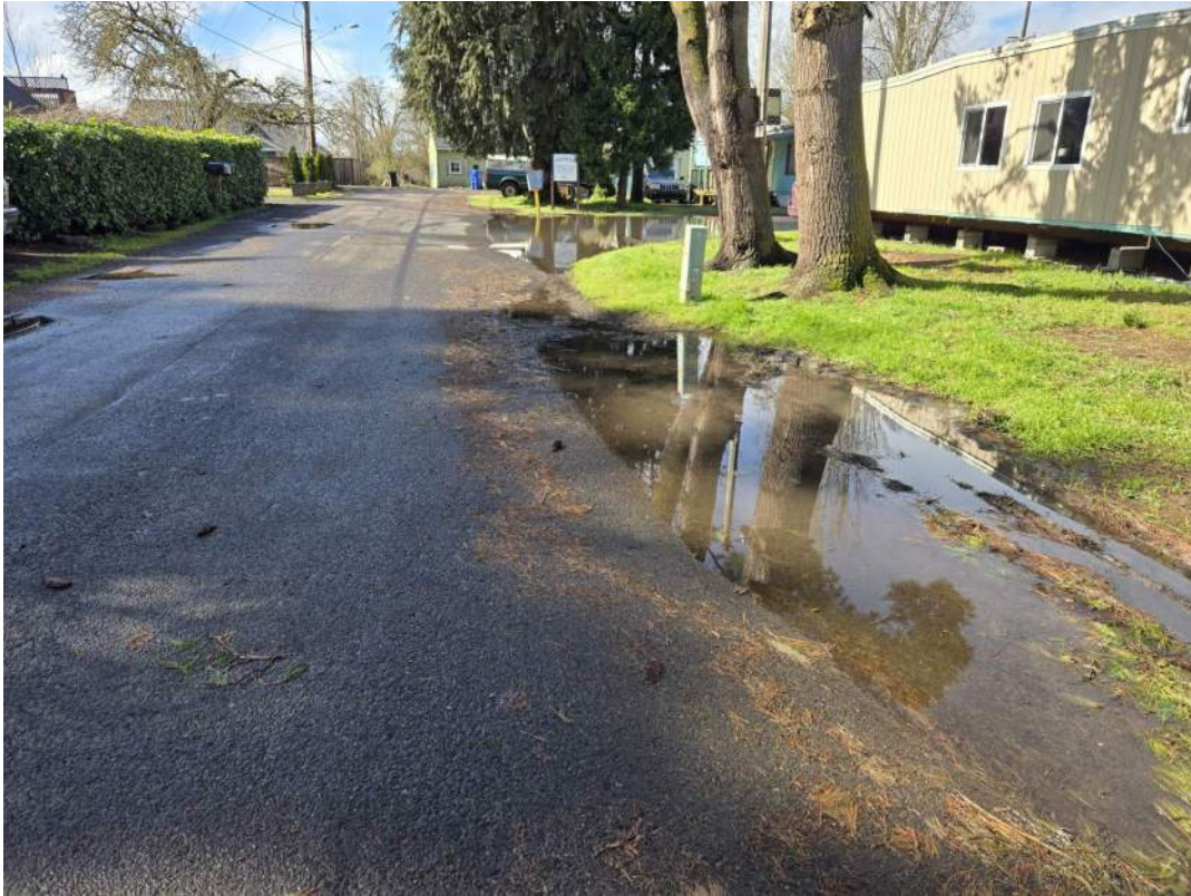
Figure 67: W. Dixon St. at Pioneer Mobile Home Park pavement in 2024.
