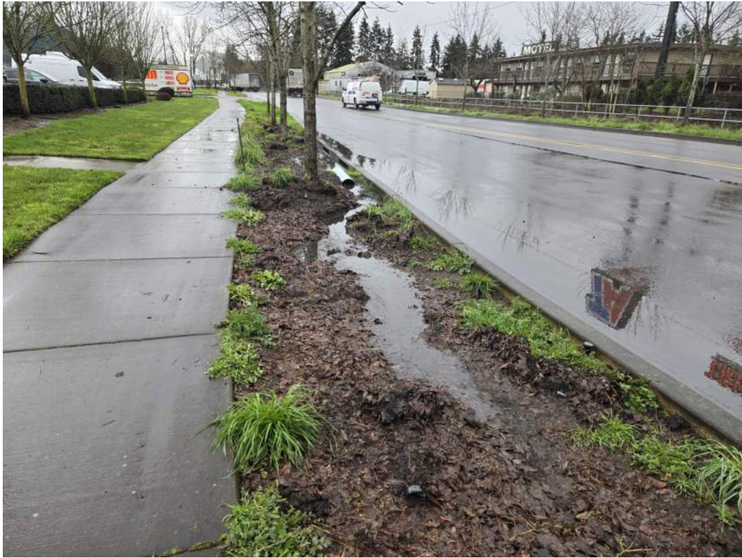
Figure 91: Coburg Industrial Way curb infiltration swale in 2024.
