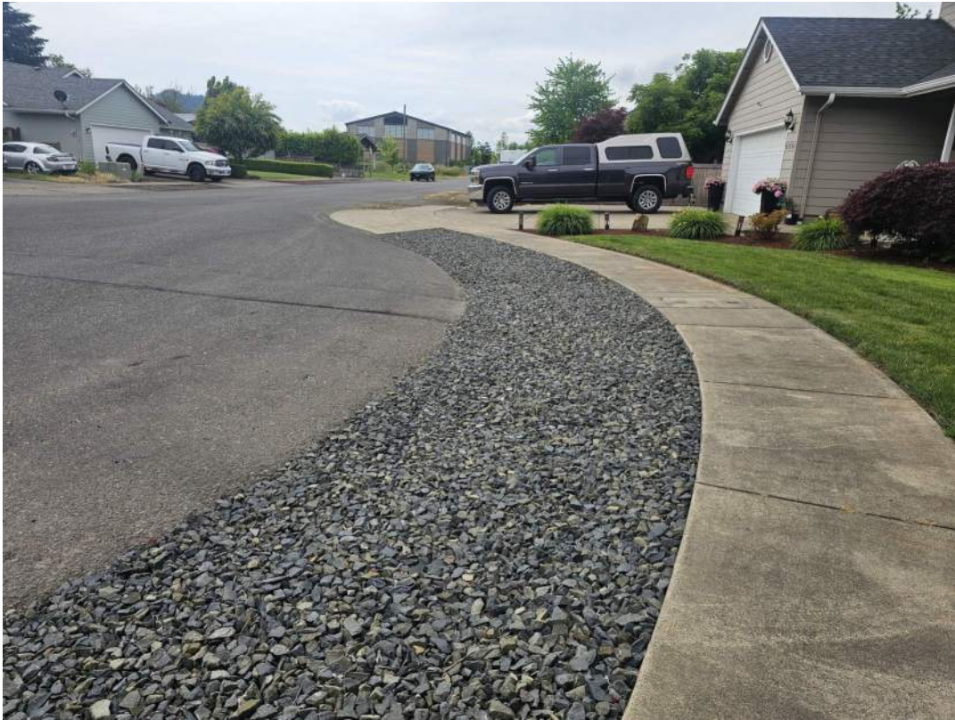
Figure 46: Reconstructed infiltration trench in 2024 on Shane Ct.
