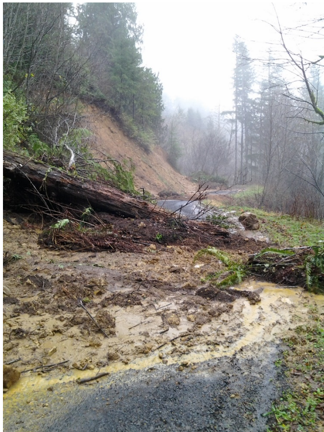
A landslide washes out a section of road near the Siuslaw River in 2014
