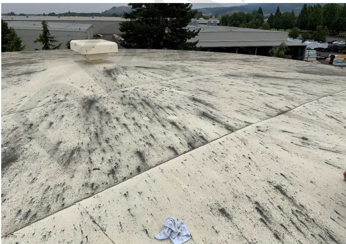
Photo 8 – Tank Exterior Roof
