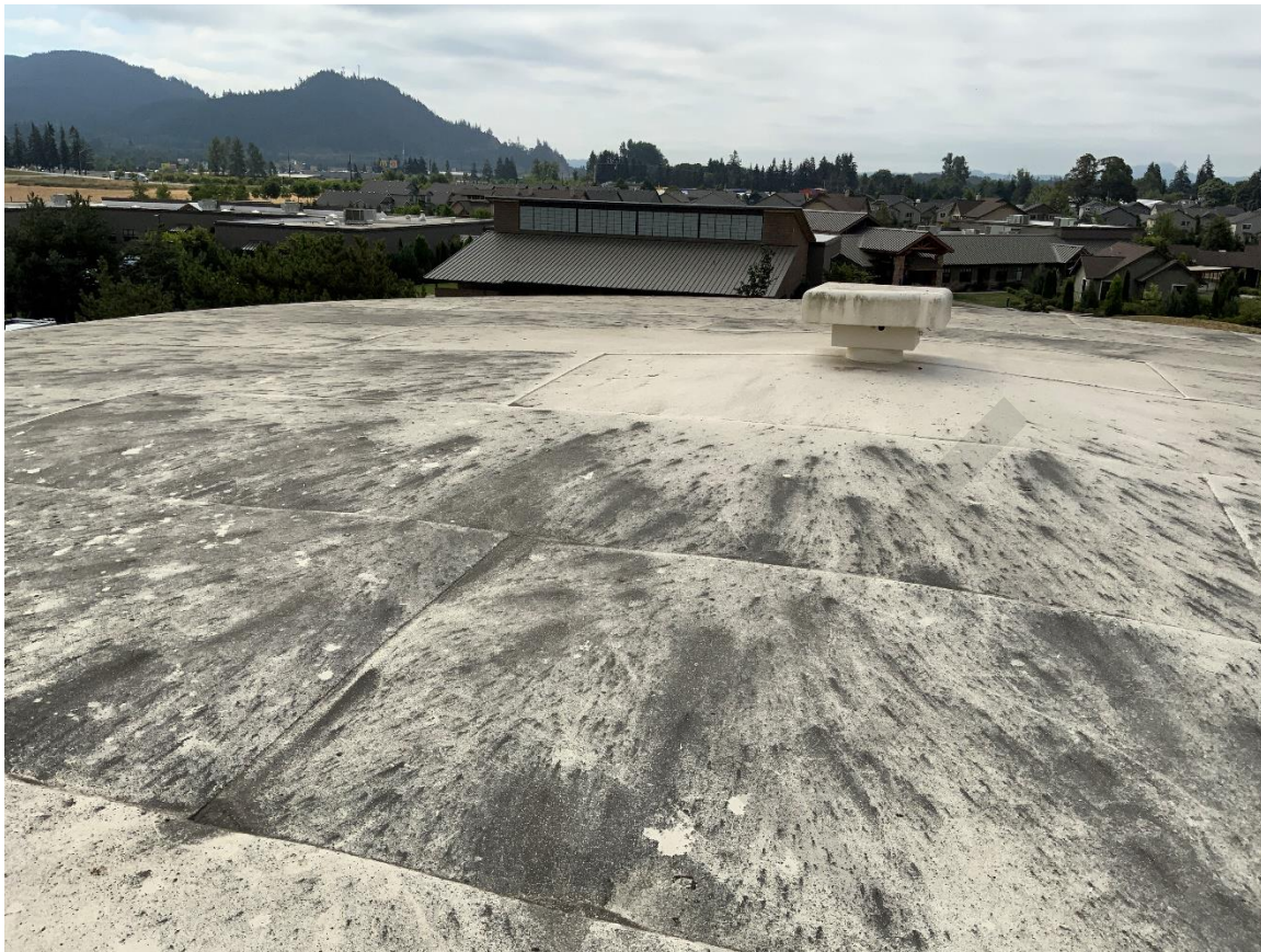
Photo 21 – Tank Exterior Roof
