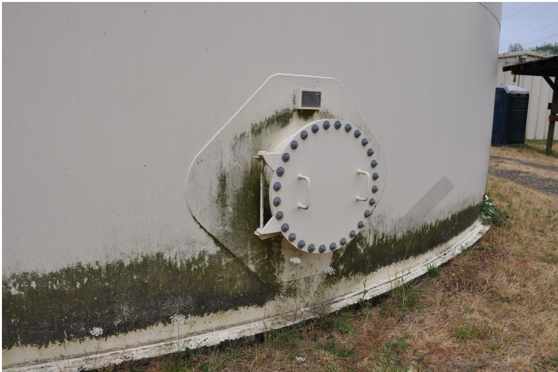
Photo 5 – Tank Exterior Hatch
