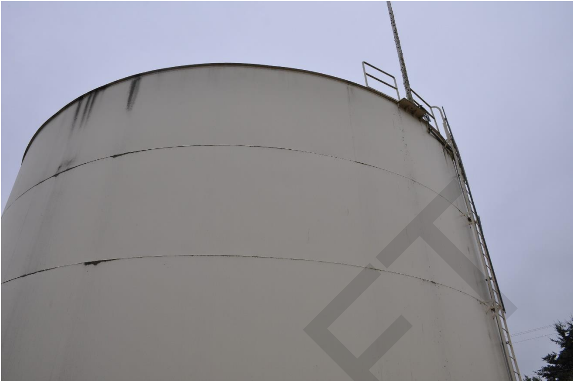
Photo 16 – Tank Exterior Upper
