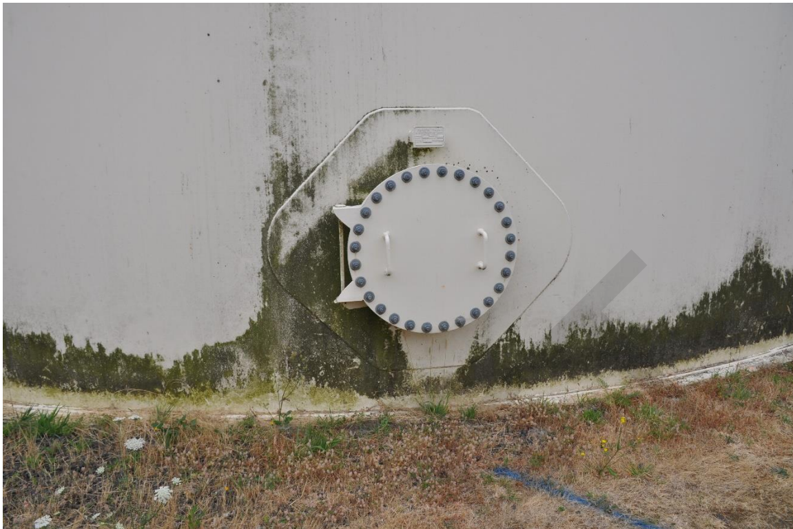
Photo 18 – Tank Exterior Hatch
