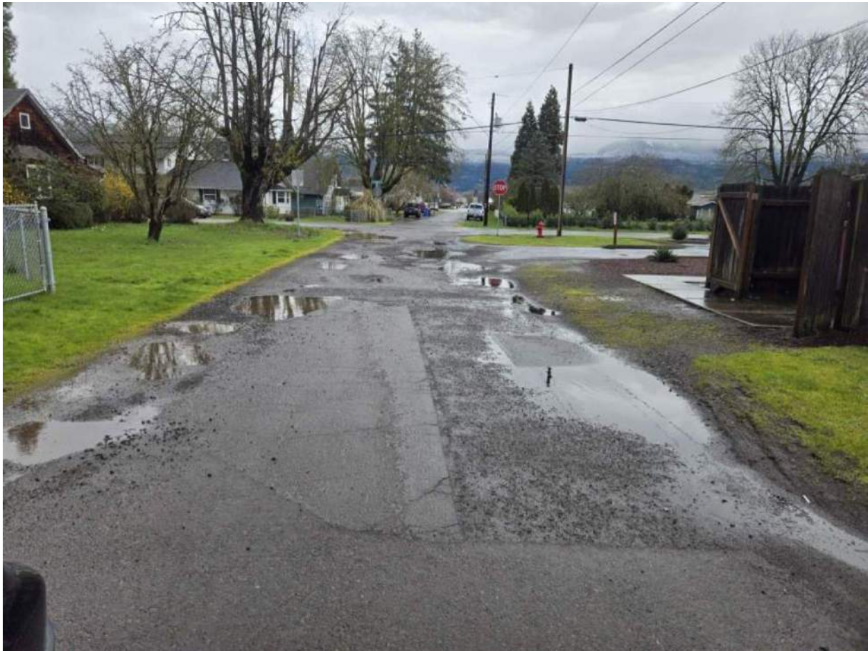
Figure 4: E. McKenzie St. between N. Coleman St. and N. Skinner St. showing degraded pavement and resulting ponded water after a mild rainfall event.
