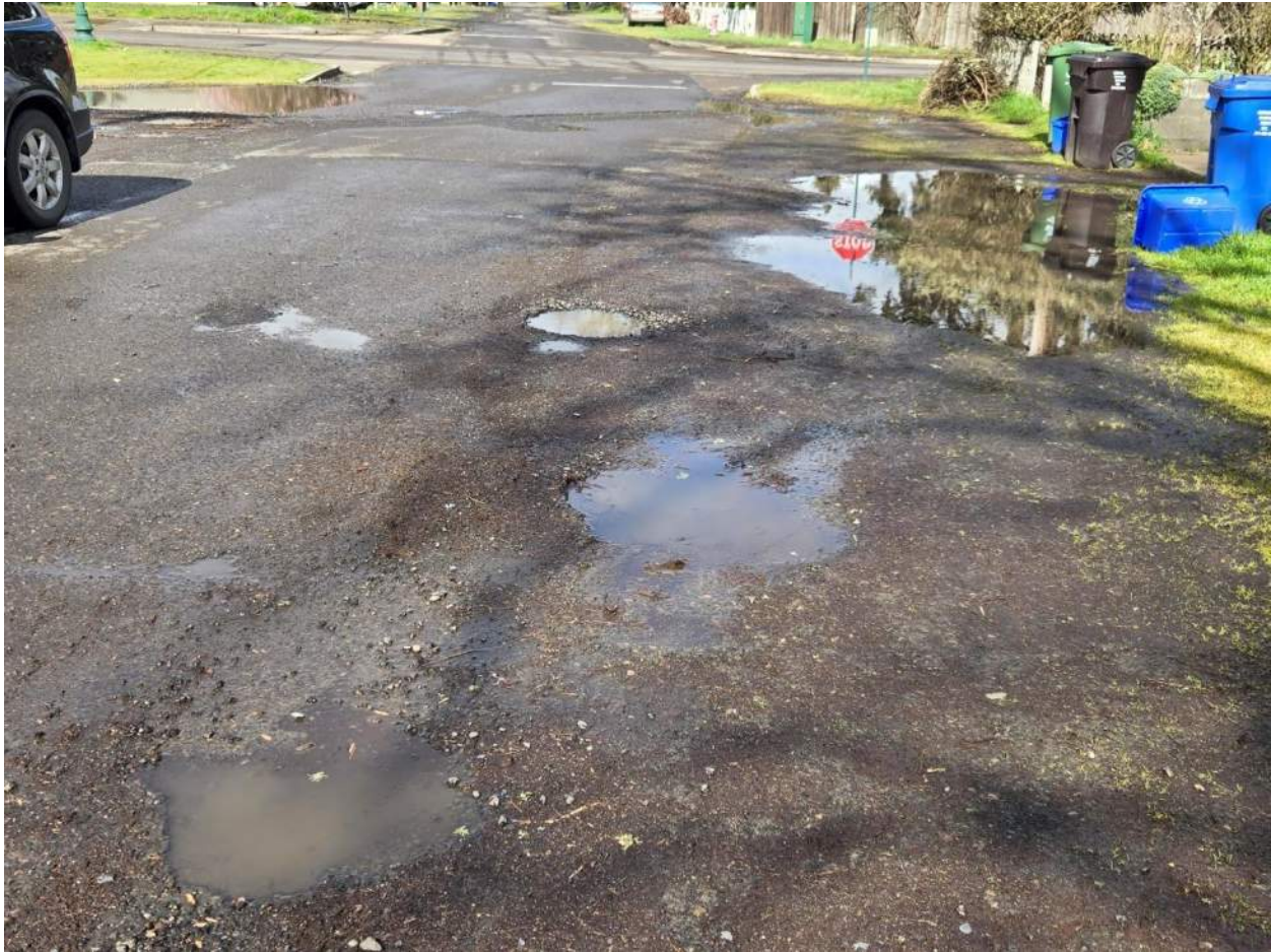
Figure 5: S. Skinner St. just south of E. Pearl St. showing roadside ponding and pavement distresses.
