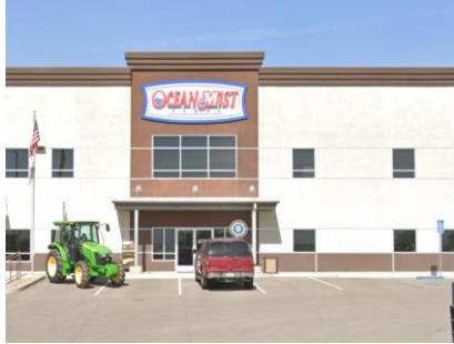
Figure 1 - 2019 Approved Main Building
