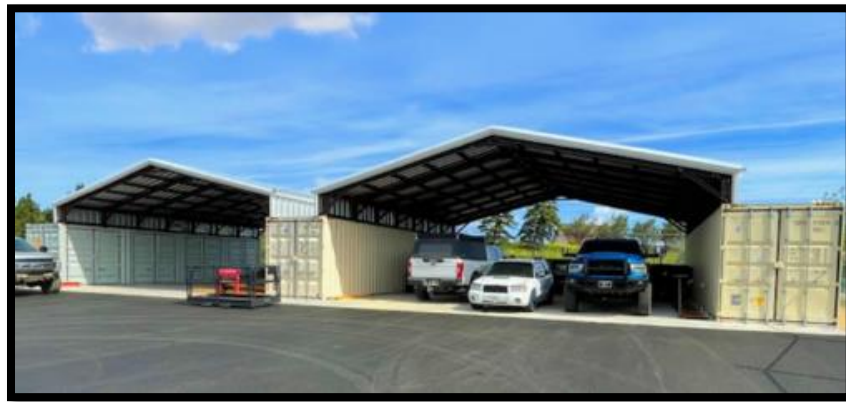
Figure 6 – Front Elevation of Eberhard Maintenance Building
