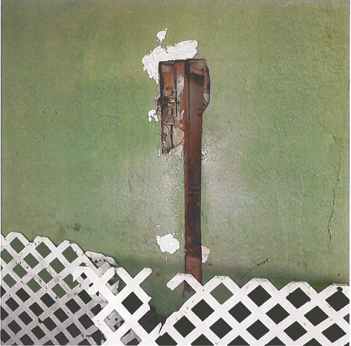
Photo #1 – Exterior Wall Saw Cuts
