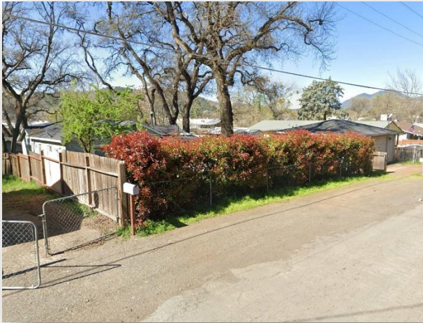
Northeast Elevation-View to the West
