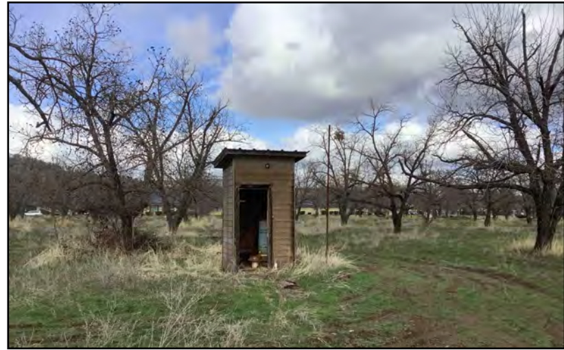
Photo 8. Photo of foundations from old residential development and large oak trees. Photo taken January 29, 2021, facing west-northwest.
