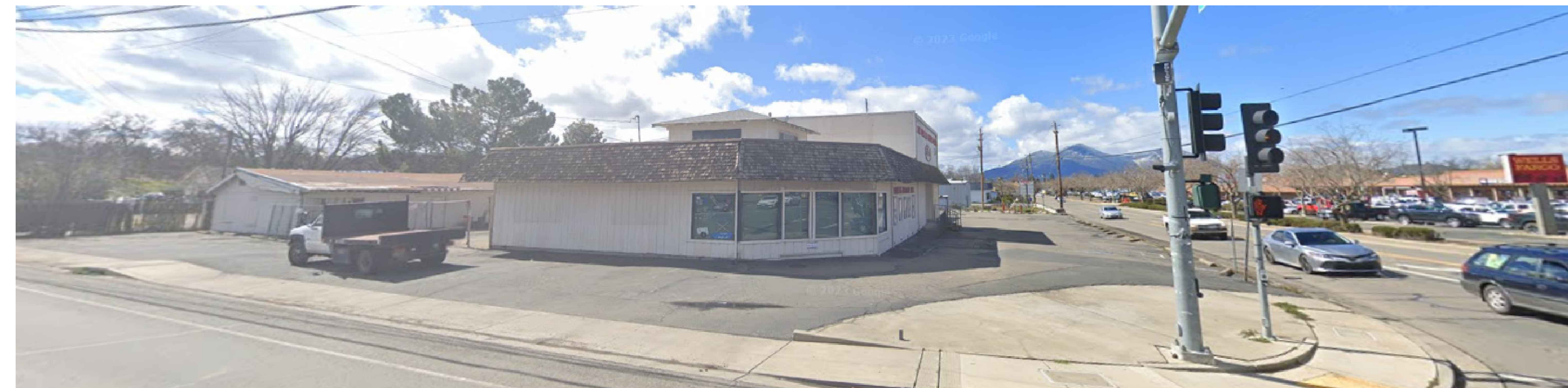
CORNER VIEW @ OLD HIWAY 53 AND OLYMPIC DR.
