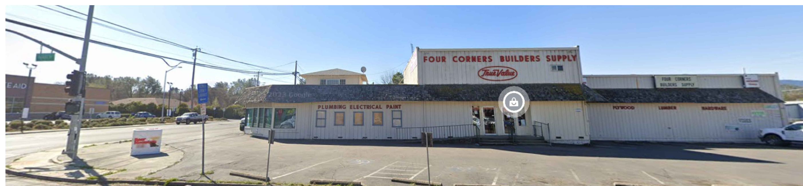
CORNER VIEW @ OLYMPIC DR. AND OLD HIWAY 53
