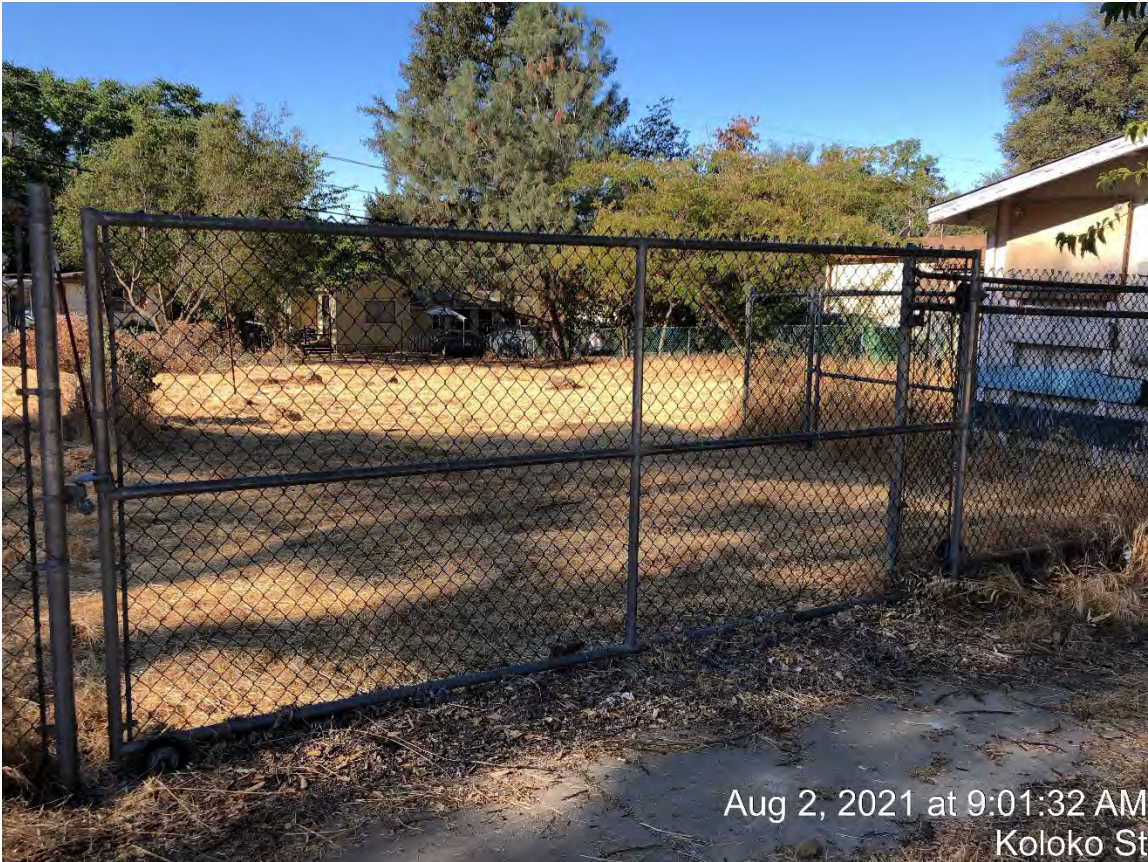
View 17: Looking southwesterly, towards the southwestern corner of project site. Lupoyoma Street beyond.
