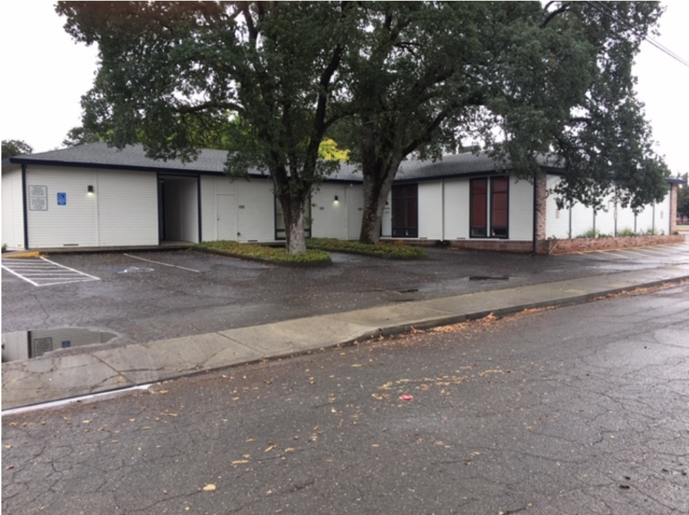
Photo No. 2: Southeasterly view of project building and site from across Emerson.
