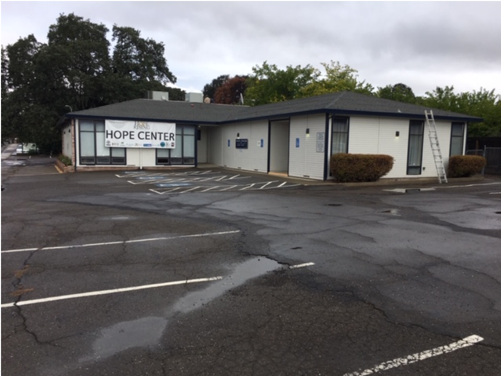
Photo No. 1: Northeasterly view project building and site from the intersection of Emerson and Olympic
