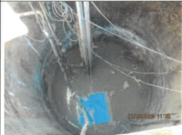
Photo 13: A photo of the north wet well at Pump Station No. 2 showing minor debris, trash, and staining on the walls.
