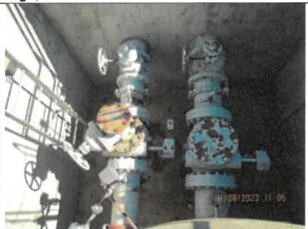
Photo 4: A photo of the one of the uncovered dry wells with minimal debris and paint chippings.
