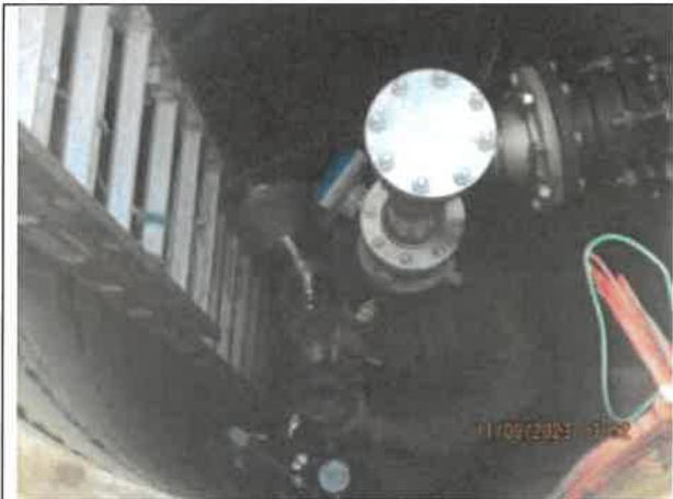
Photo 28: A photo of the direct in-line pumping system being put into place at Pump Station No. 6.
