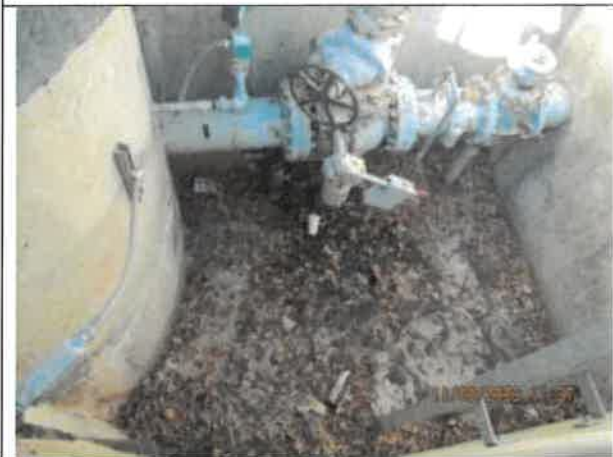
Photo 11: A photo of the uncovered north dry well at Pump Station No. 2 showing debris and minor trash.
