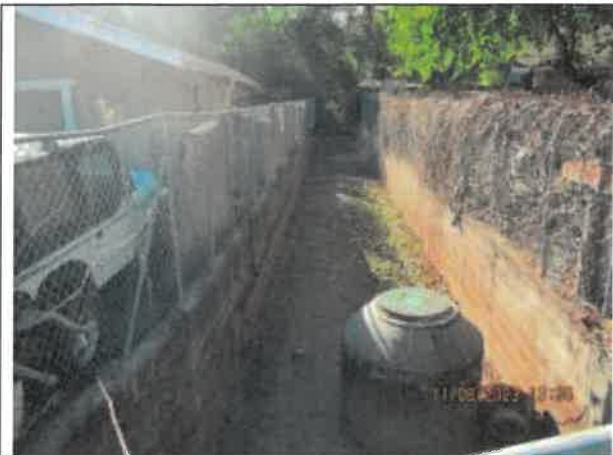
Photo 27: A photo of the manhole in the canal on Stonybrook Drive.
