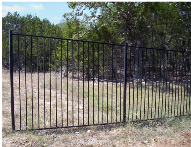
Figure 1, Wrought Iron Fencing:
