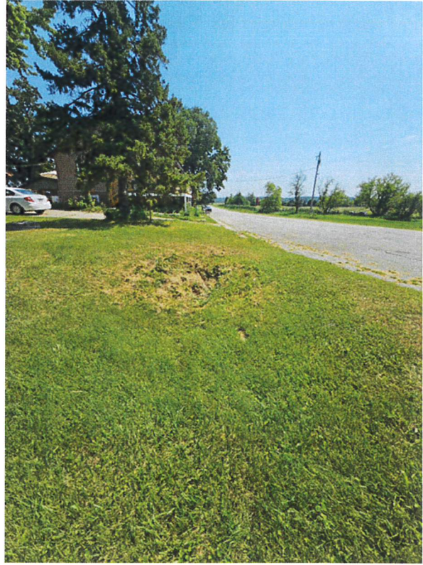
▲ 6 – West End of Winnegamie Drive Culvert (North Side) Upstream End of Bennett’s Auto Culvert
