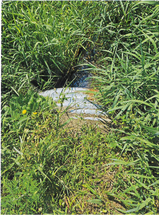
▲ 1 - Culvert on South Side of Winnegamie Drive
