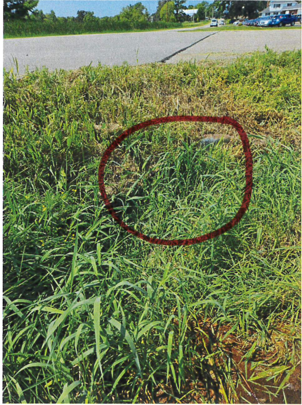
▲ 2 - Culvert at Northeast Corner
