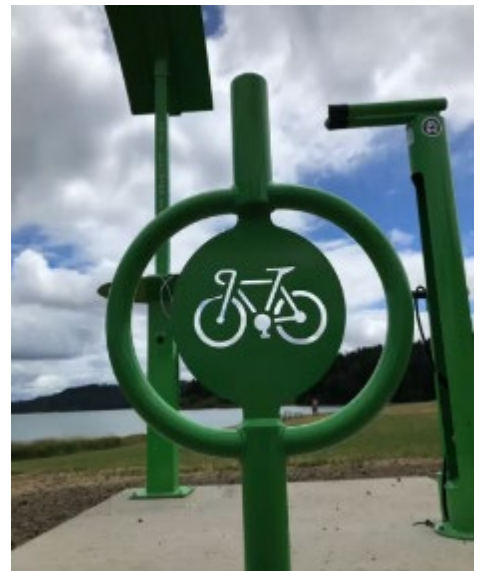
Bike parking, fix it station, and solar charging at Hagg Lake (source: Washington County Parks)
