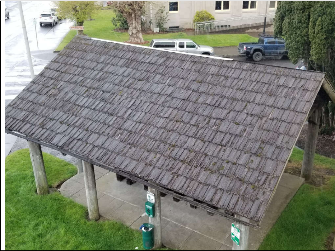
Existing Cedar Roof
