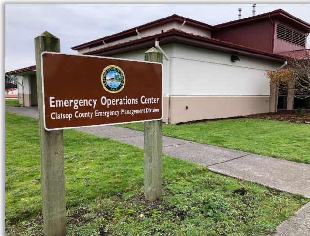
Figure 9: Clatsop County Emergency Operations Center, Warrenton, Oregon
