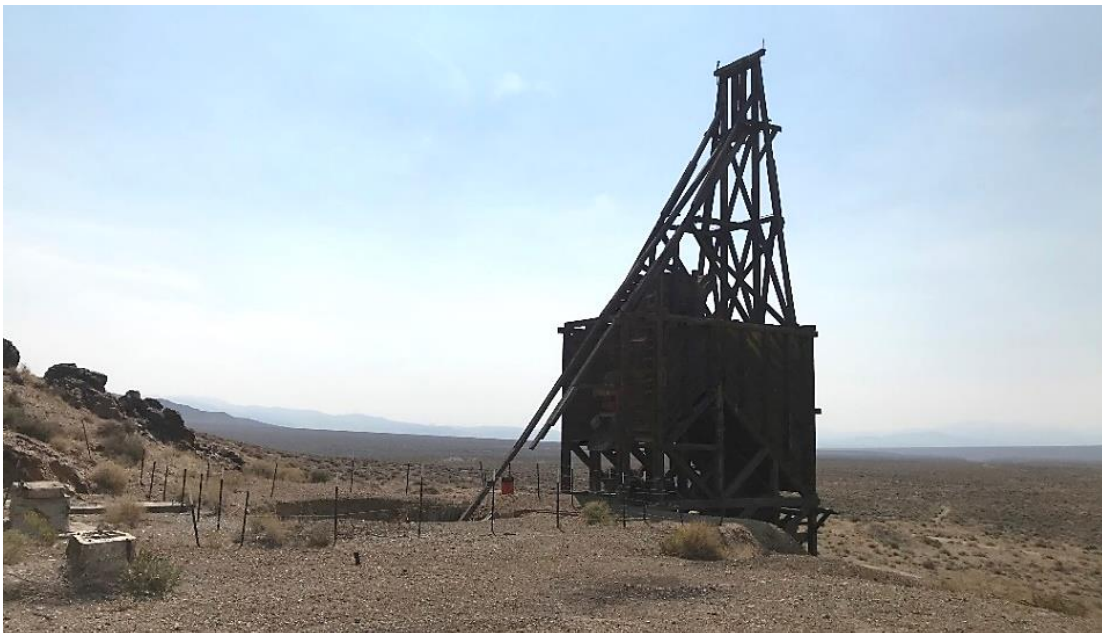
Photo 2 - Headframe at Quartz Mountain, Nye County, NV.
