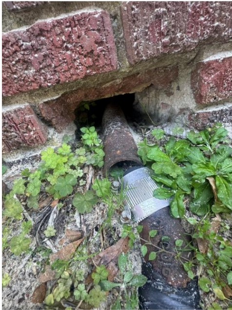
Figure 12 – Disconnected and/or Abandoned Pipe
