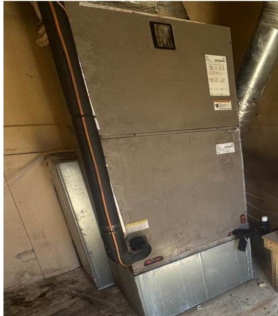
Figure 1 – Air Handling Unit (AHU-1)
