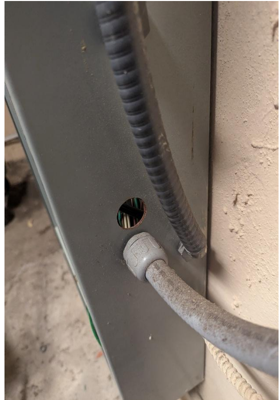
Figure 7: Exposed Electrical Gap
