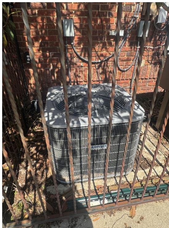
Figure 4 - Heat Pump Unit (HPU-2)
