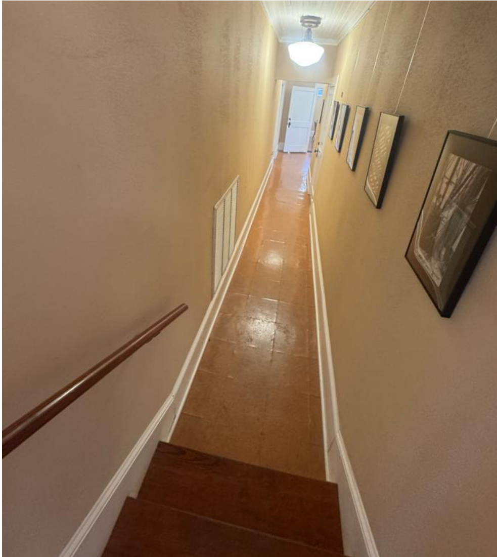
Figure 7 – Sidewall Return Grille in Corridor
