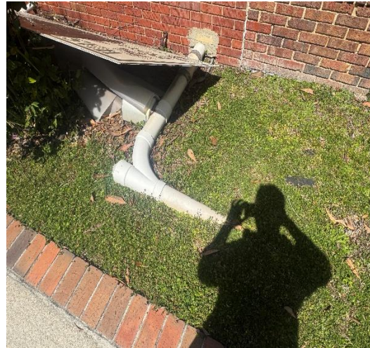
Figure 13 – Exposed Piping on Exterior of Building
