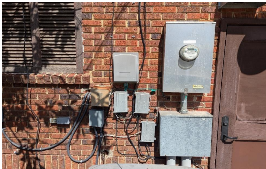
Figure 1 – Exterior Electrical Meter and Service Junction Box
