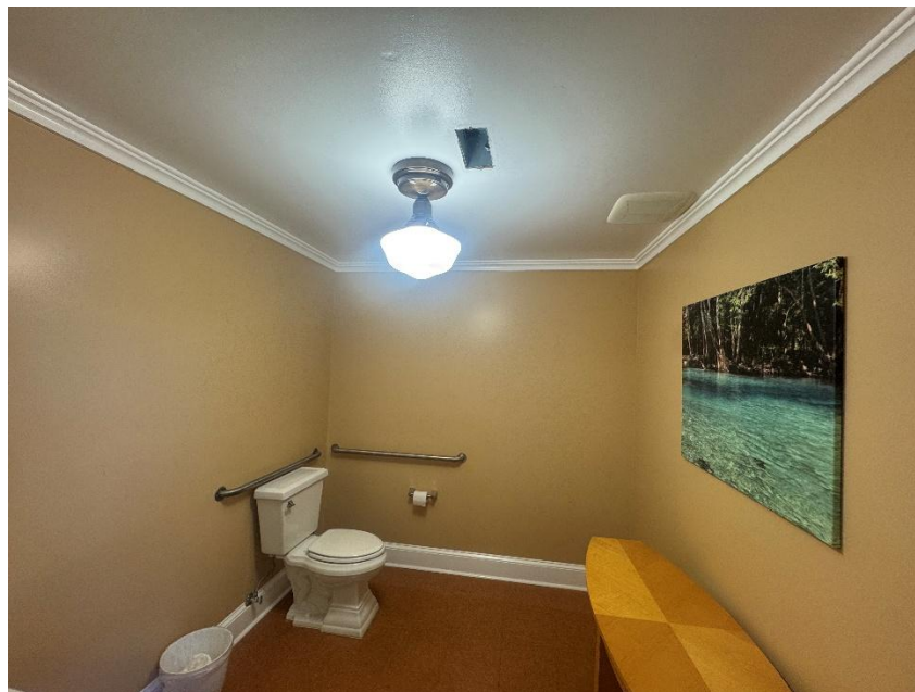
Figure 6 – Missing Ceiling Grille
