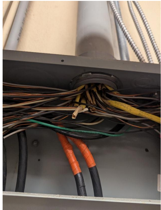
Figure 5: Abandoned cabling
