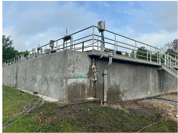
Northeast corner - Aeration Effluent Channel
