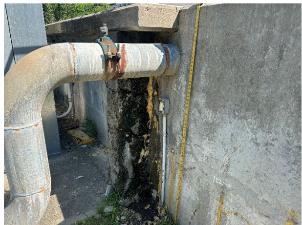
Northwest corner - Aeration Effluent Channel
