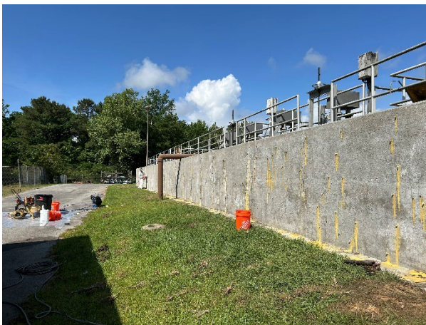
Footing Line - Aeration Effluent Channel
