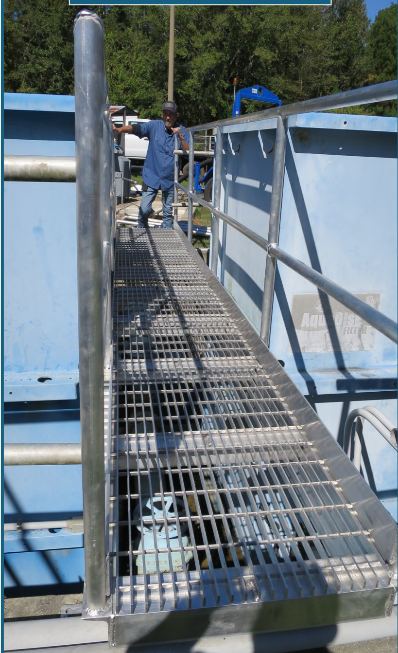
New Catwalk on Filters
