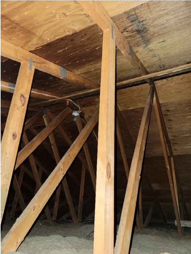
Wood Rood Trusses
