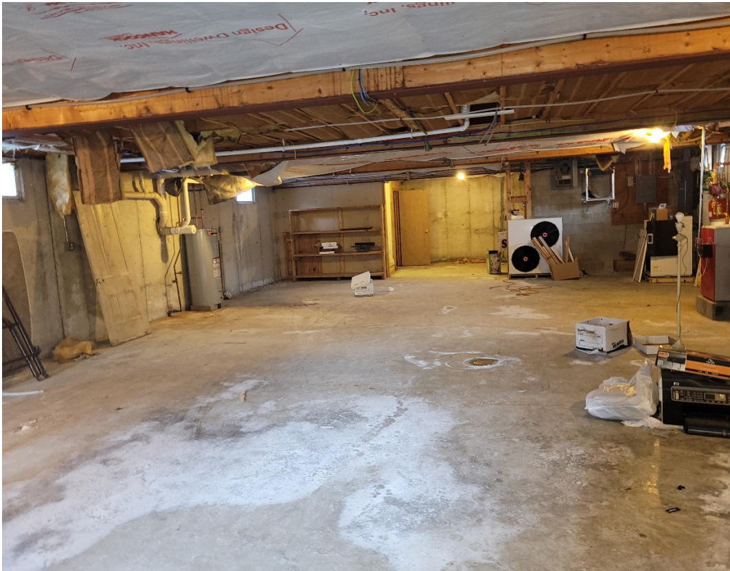
View of Basement
