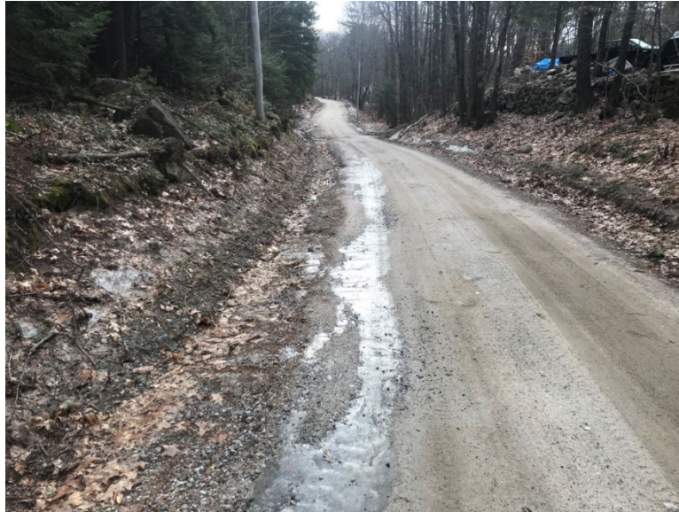
Roadside Drainage – Jim Small Road
