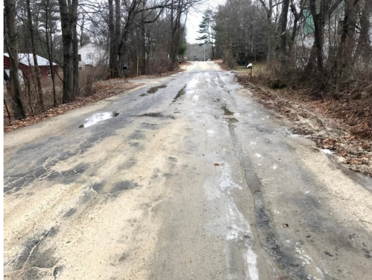
Roadside Drainage – South Casco Village Road
