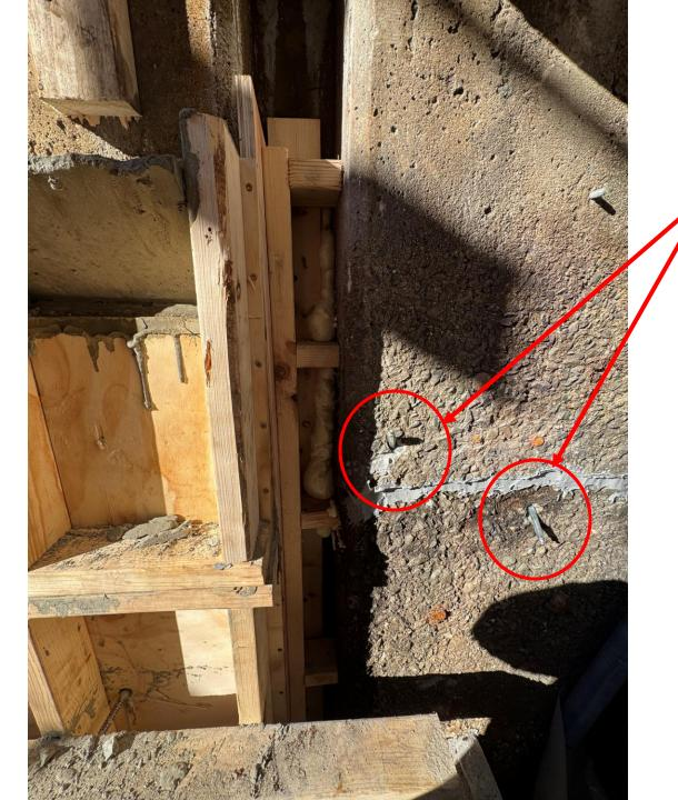
Fittings to pump high pressure polymer crack filler into small cracks
