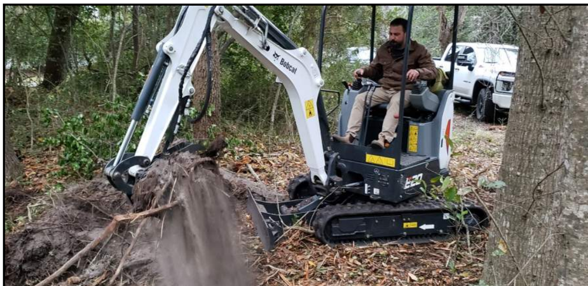
Figure 17. Excavating trench adjacent to the abandoned house structure.
