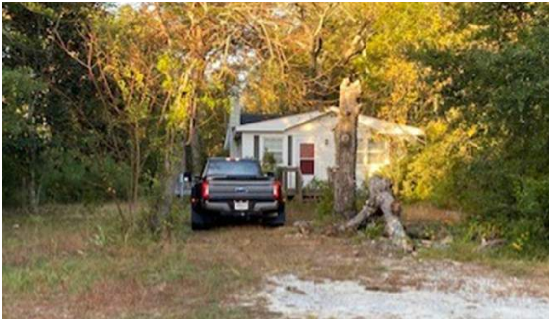
Figure 2. Abandoned house on survey property at 1215 St. Joseph Street.
