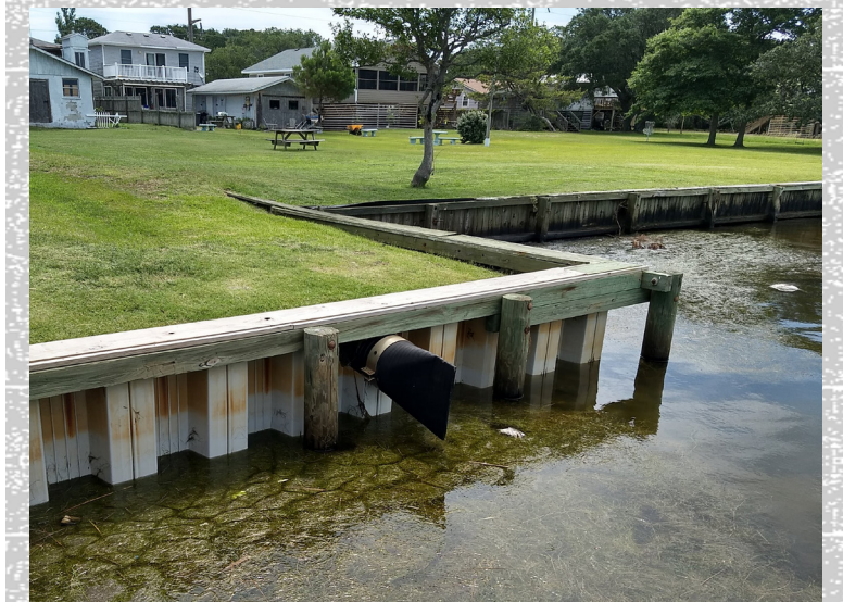
Stormwater retrofits can give temporary reprieve from sea level rise for many years.
