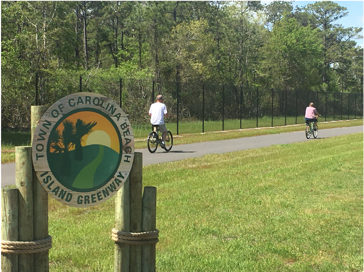
The recently constructed Island Greenway is a hit with residents and visitors
