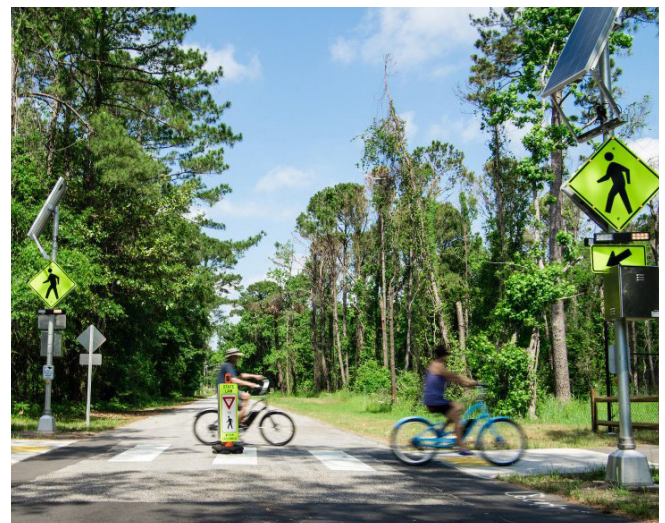
Newly installed Rectangular Rapid Flashing Beacons (RRFBs) were installed to improve pedestrian and bicycle safety and driver yielding compliance on Island Greenway crossings (Photo credit: VisitNC)
