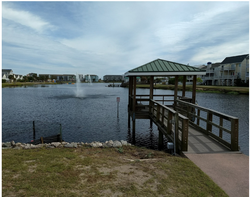
The lake was recently dredged and upfitted with larger pumps to better manage stormwater.
