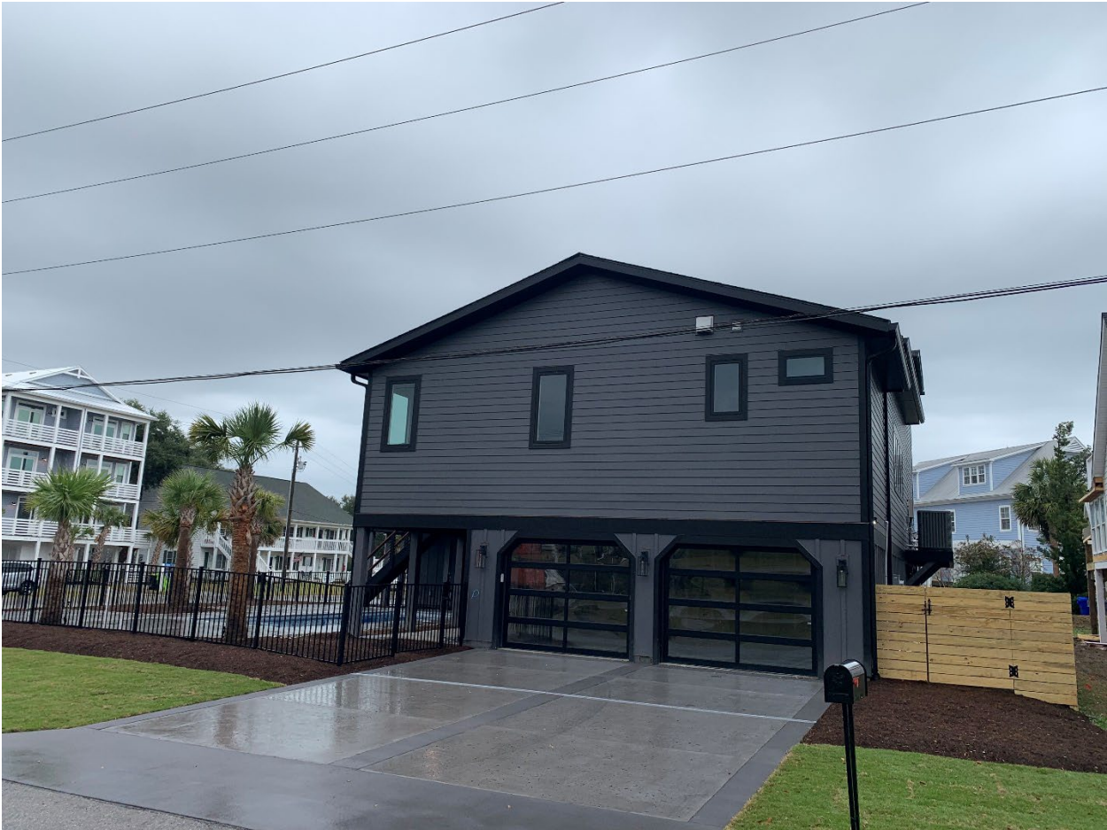
CORNER SIDE FROM DRILL SHELL LN:
