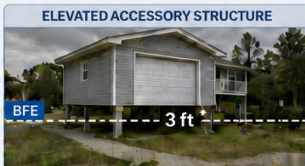
Garages and accessory structures also raised.
