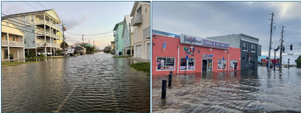
Figure 2. Representative flooding conditions in Carolina Beach, including high tide flooding in a low-lying residential area (left) and rainfall flooding affecting a commercial corridor (right). These examples illustrate the range of coastal and stormwater flooding challenges that affect community access, infrastructure performance, and overall resilience. Photo credits: Tommy Horn (left) and Suzi Drake (right).
