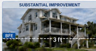
Raised to meet 3 ft freeboard standard.
