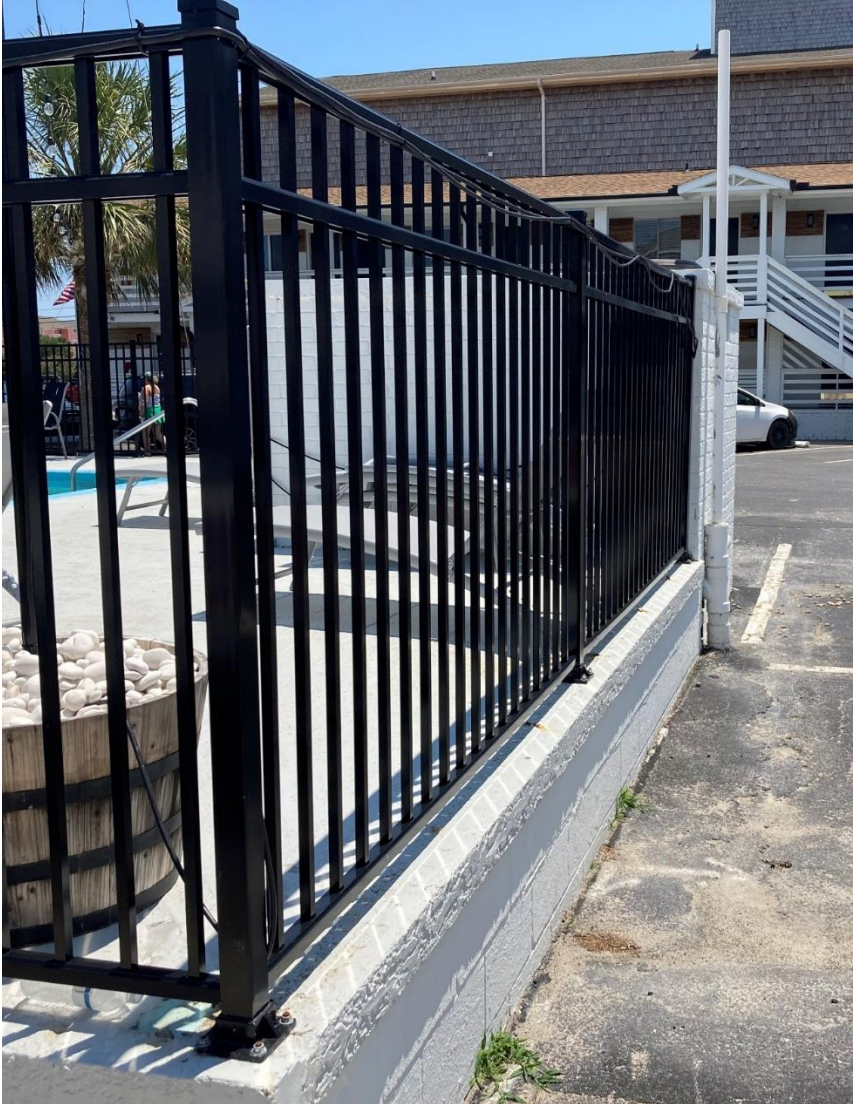
Current Fencing Compared to Brick Pump House
