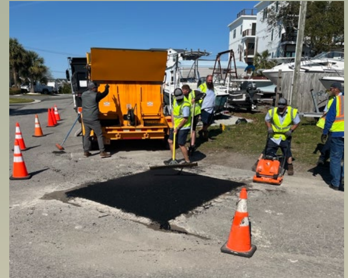
Training and implementation of Town conducted asphalt patching program
