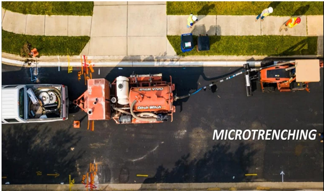
Figure 4: Trench in pavement (Microtrenching)
